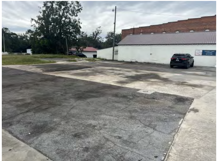
PHOTOGRAPH 2 View of the west portion of the subject property, facing southwest.
